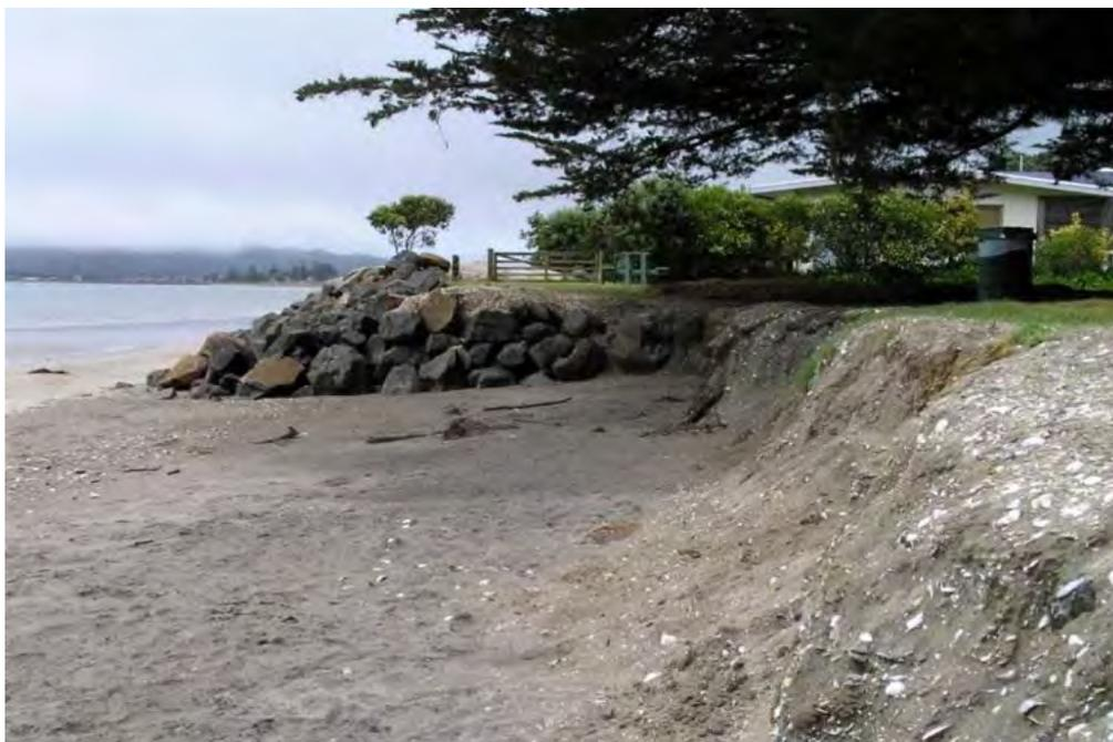
**Figure 10-1: Erosion beside a sea wall in Whitianga. Photo: R. Bell, NIWA.**
